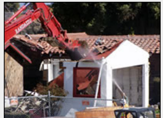
Photo: Construction on Hidden Court Motel
